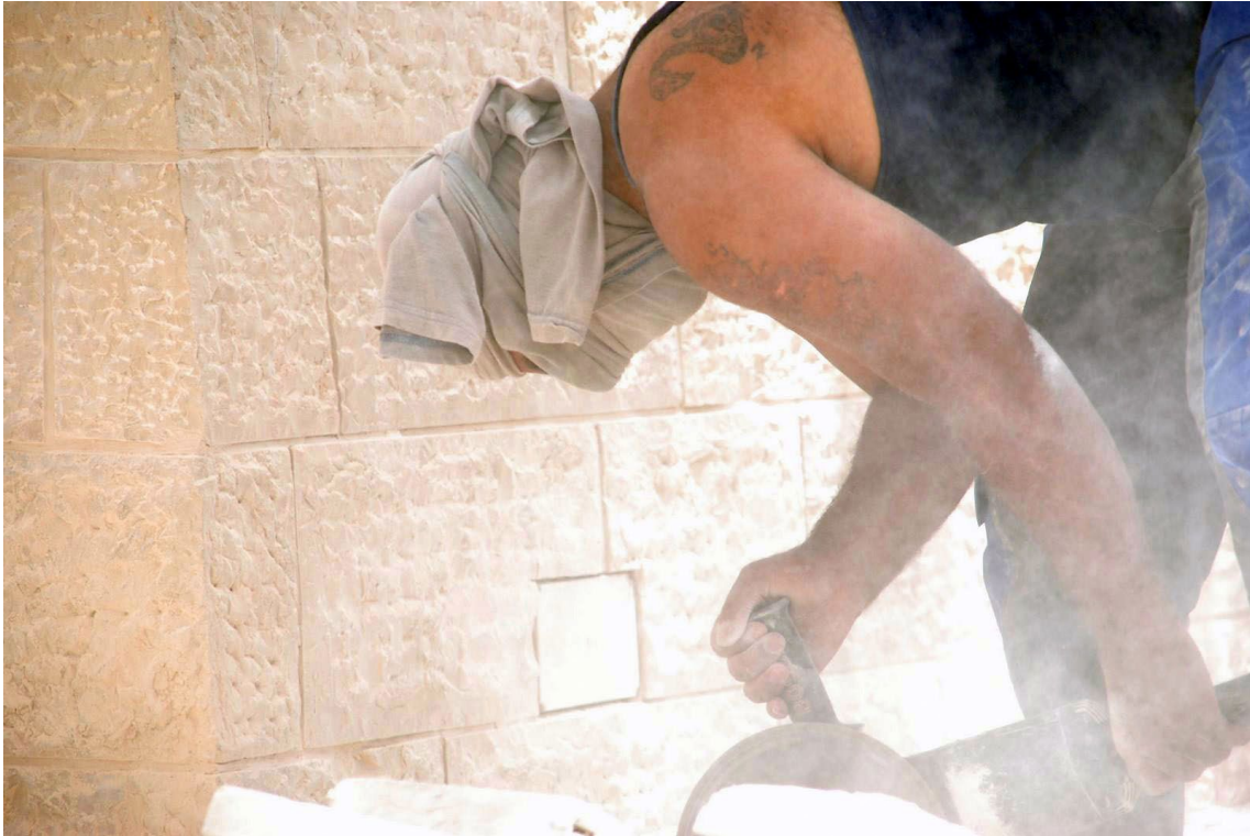
Palestinian workers face unsafe conditions in Israel's construction industry. Photo: ILO
