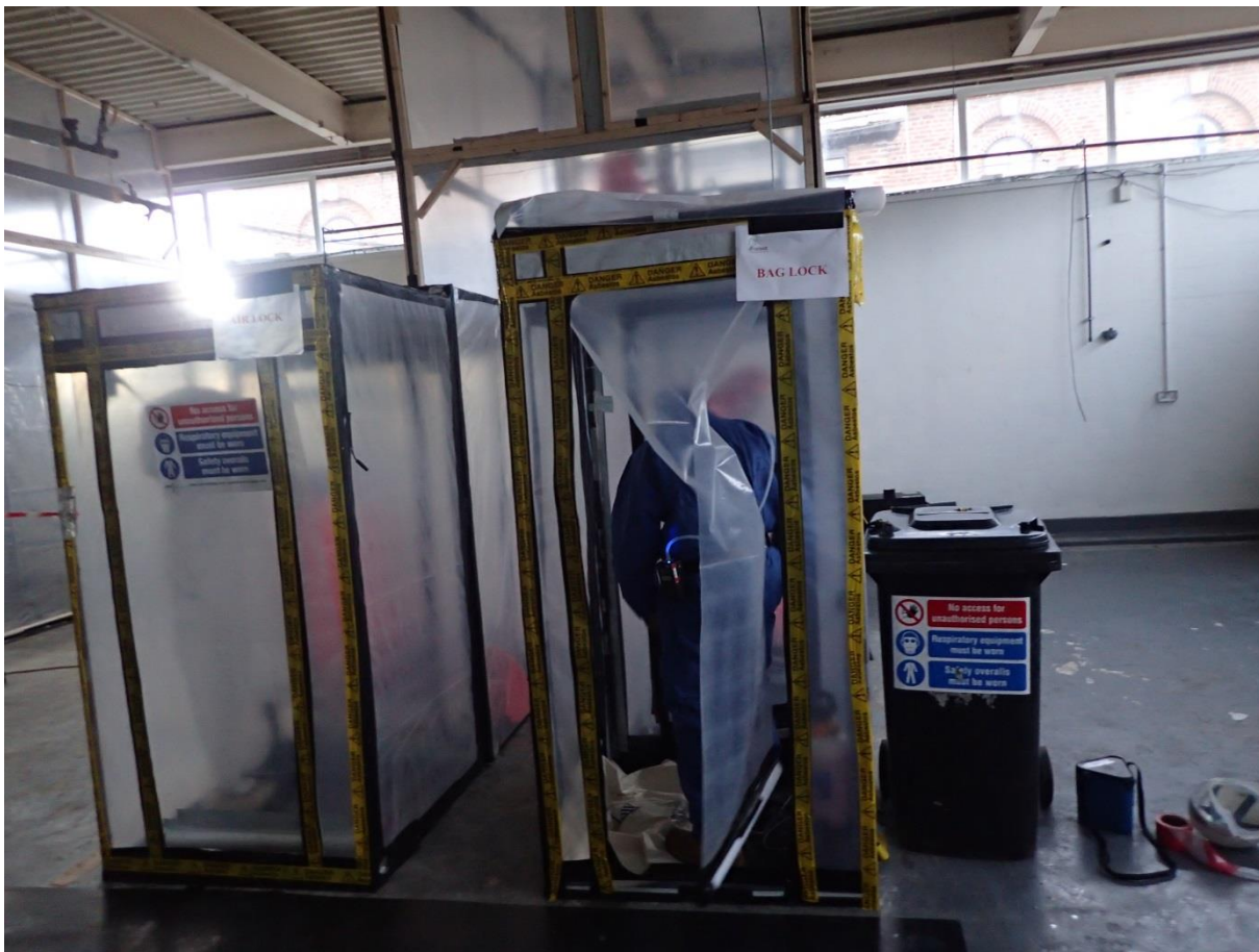
Figure 2. An asbestos removal worker wearing a sampling pump whilst removing waste from an enclosure
