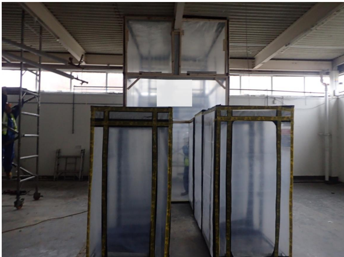
Figure 1. An asbestos removal enclosure with airlocks being constructed on a site visited by HSE scientists
