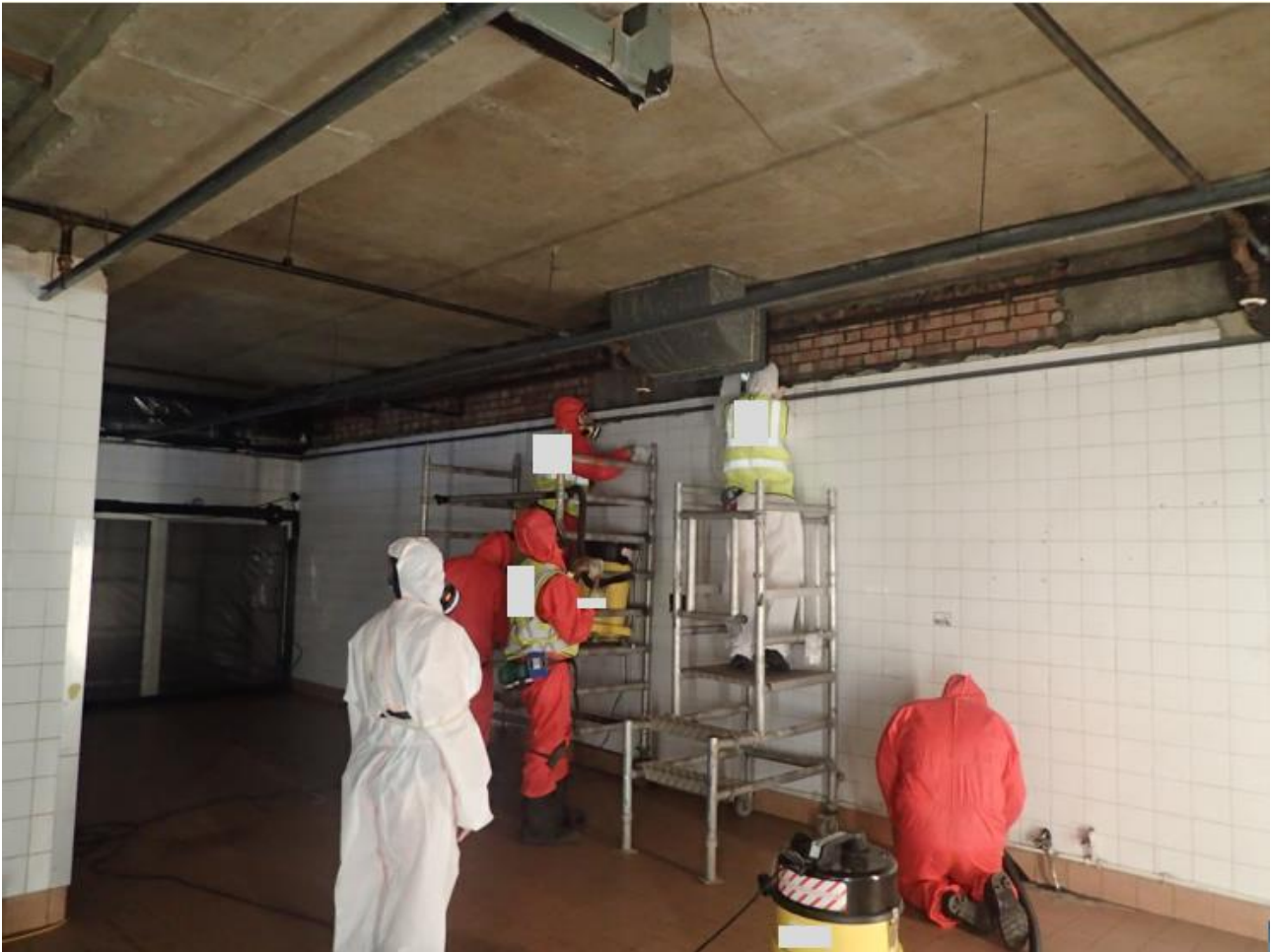
Figure 3 Analyst and trainees (white coveralls) carrying out visual inspection accompanied by removal workers
